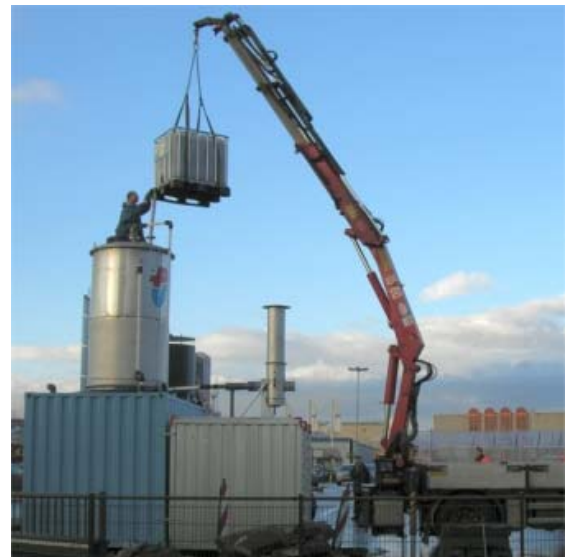
Filling the reactor with anaerobic sludge in December 2005
